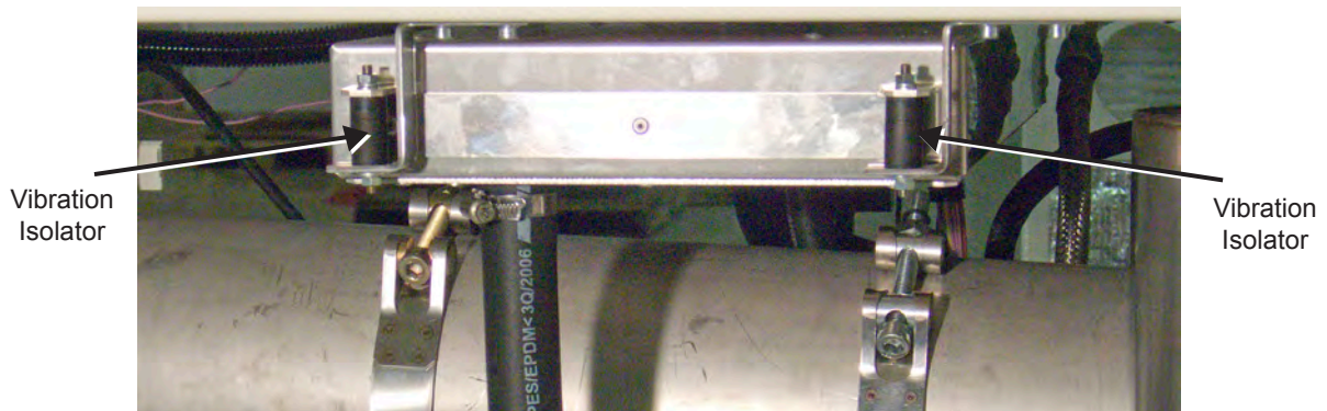
Figure 2.11 Air Intake Damper Vibration Isolators
